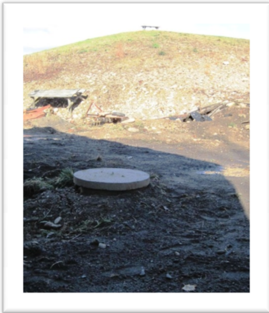
A beautiful blossom: the new septic tank
